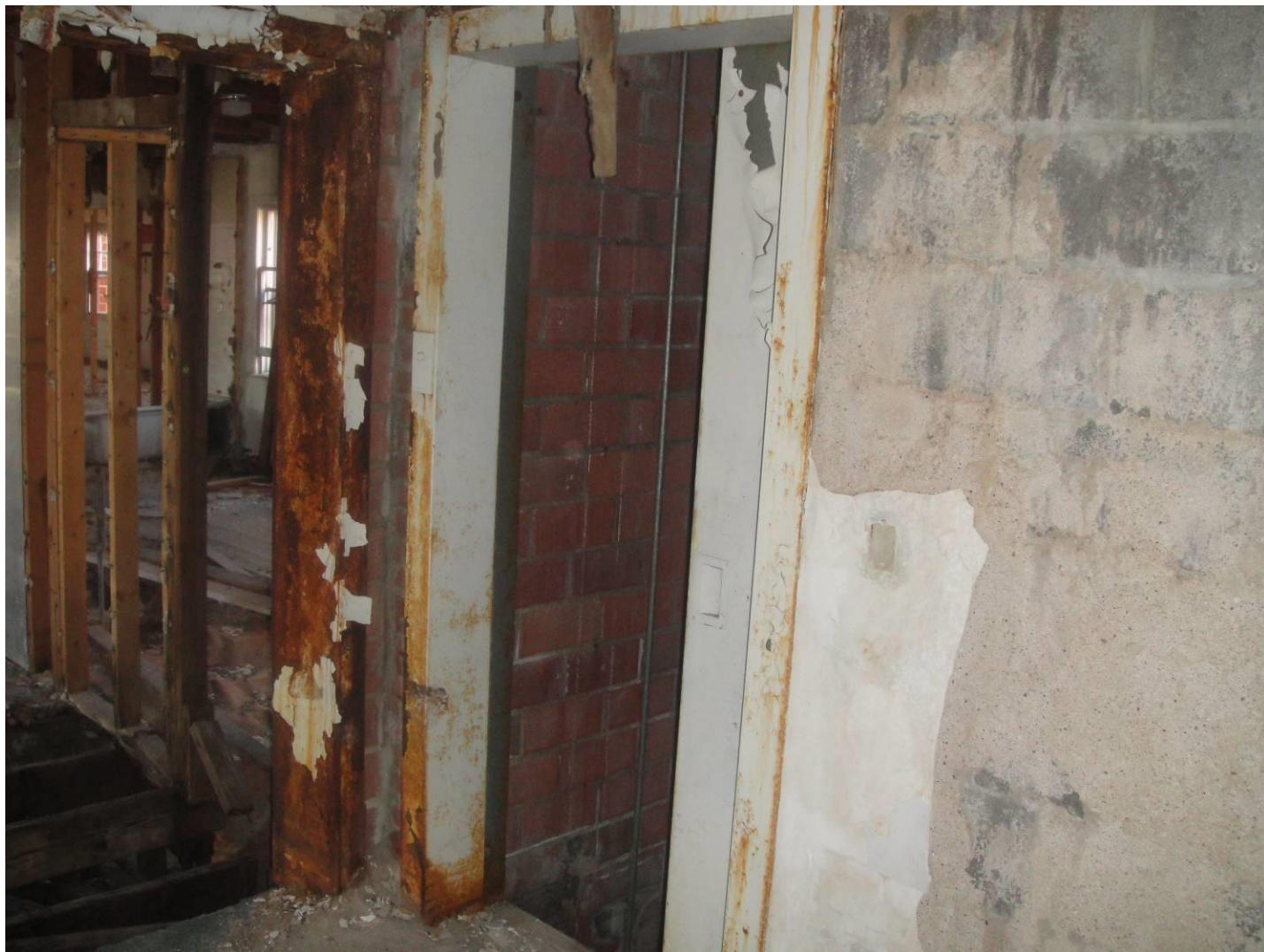
Photo 15— View of elevator location. Elevator is out of commission and door is ajar and unsecured. Condition presents an unsafe environment which may lead to a fall hazard into the basement elevator pit.
